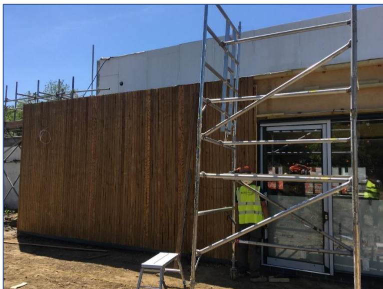
Exterior cladding being fitted
