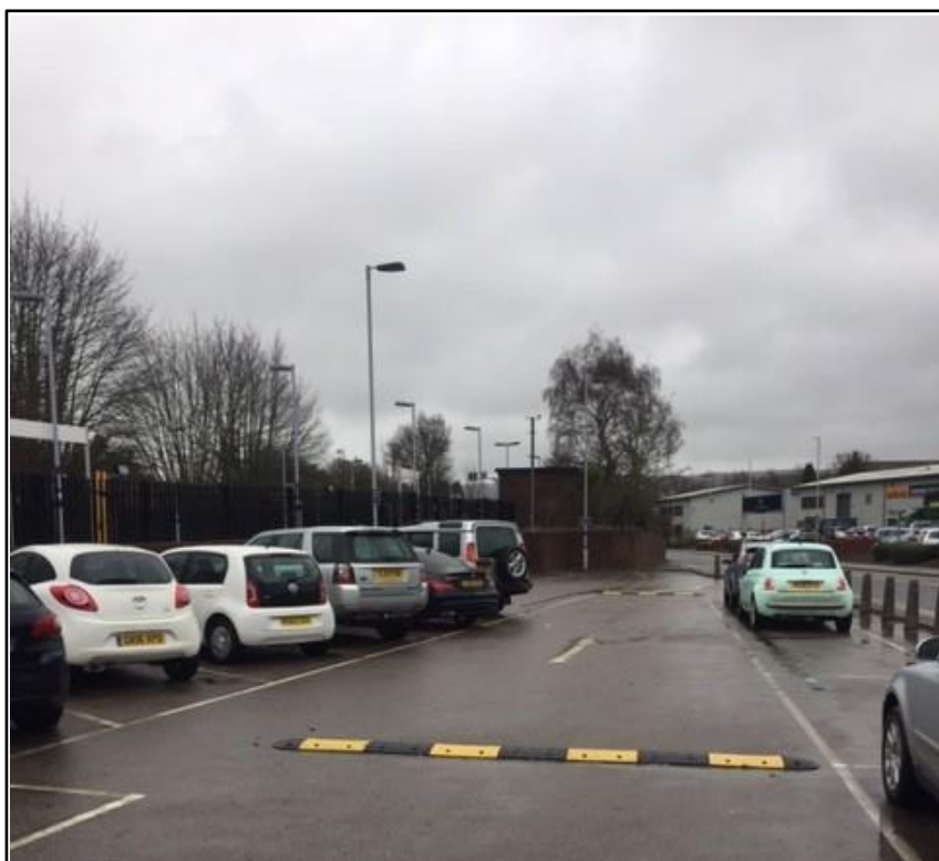
Image 2. The station car park with the brick relay room in the background
