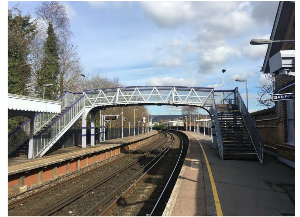
Plate 8: Bridge across platforms to the west
