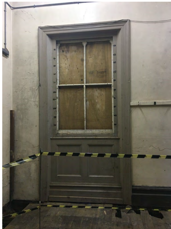
Plate 22: Typical internal joinery detail
