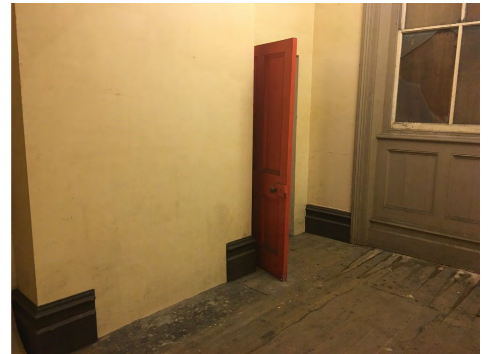
Plate 17: Interior view within the 'Ladies Waiting Room'
