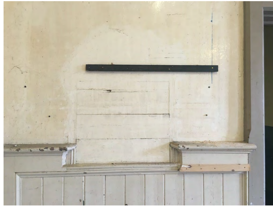
Plate 19: Boarded up ticket window as seen from the main booking hall
