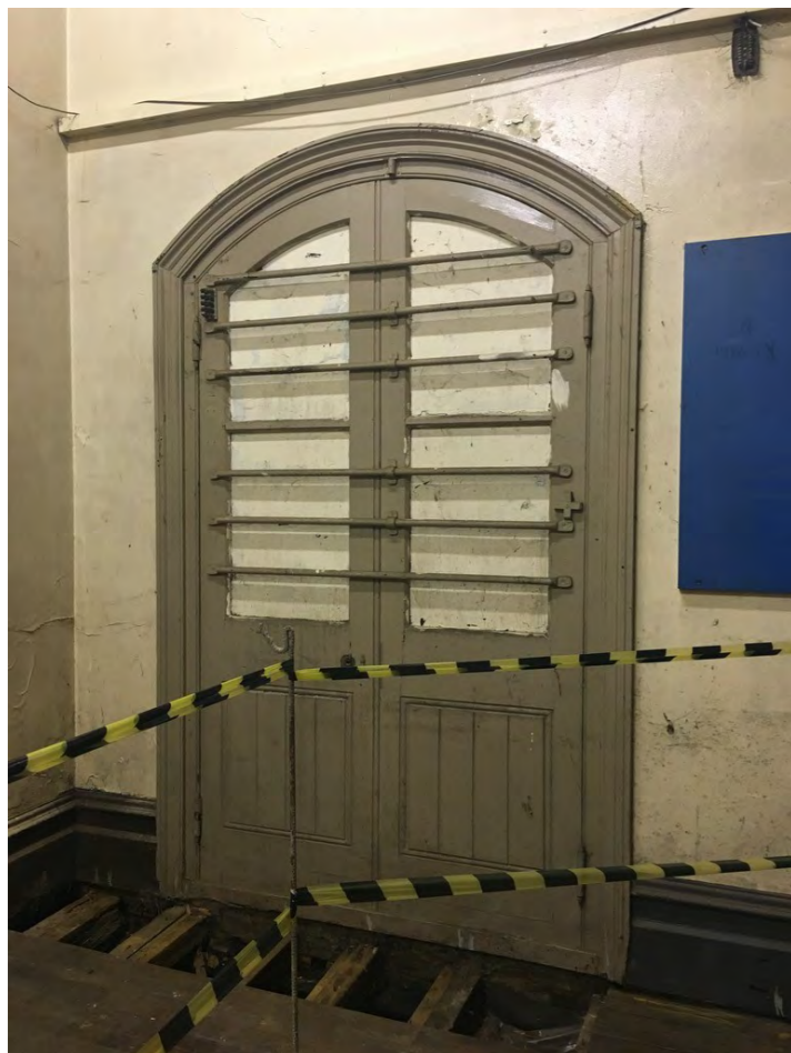
Plate 21: Typical internal joinery detail
