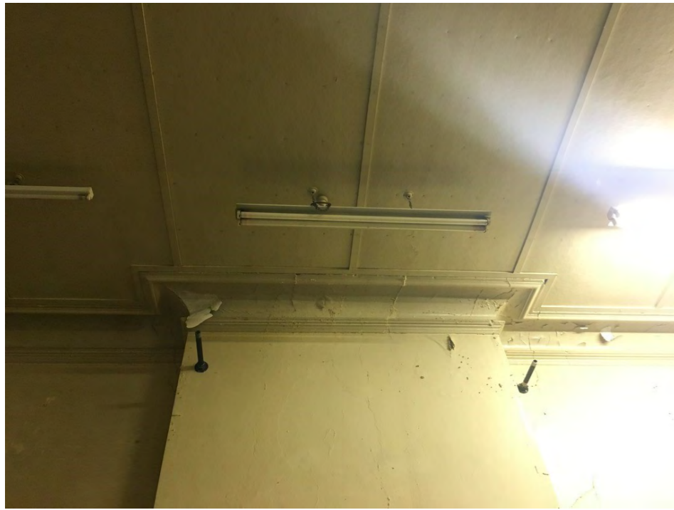
Plate 18: Typical cornice within the 'General Waiting Room'
