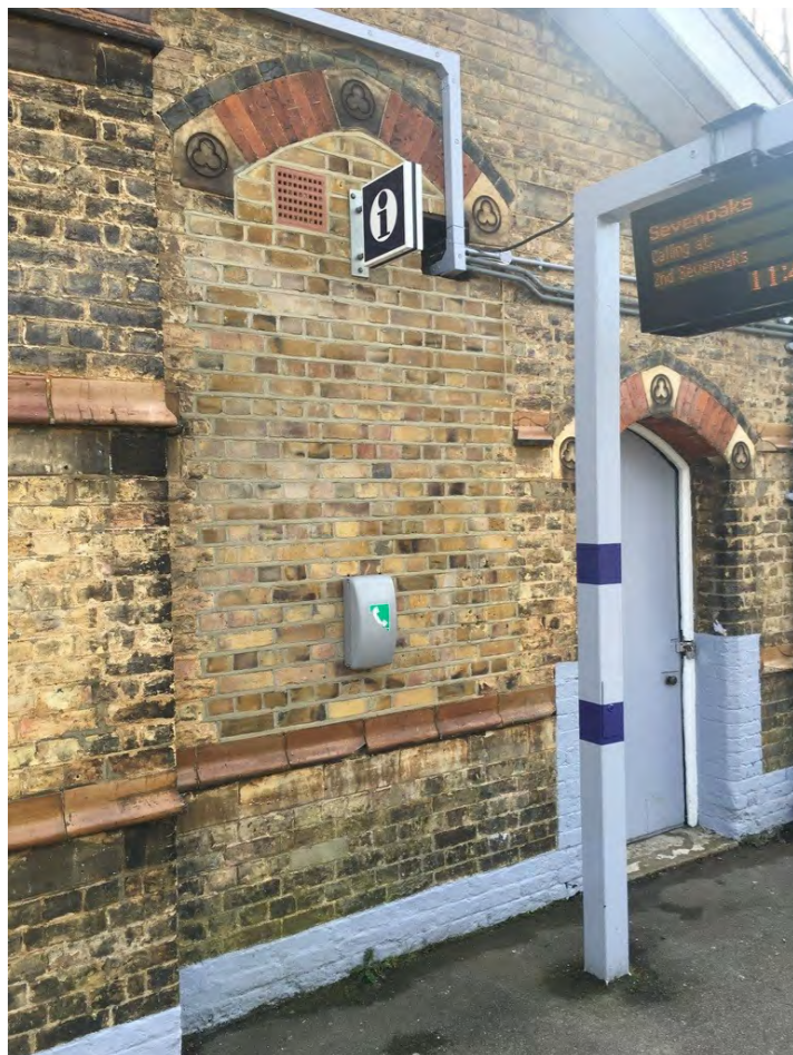
Plate 9: Alterations present to the west elevation
