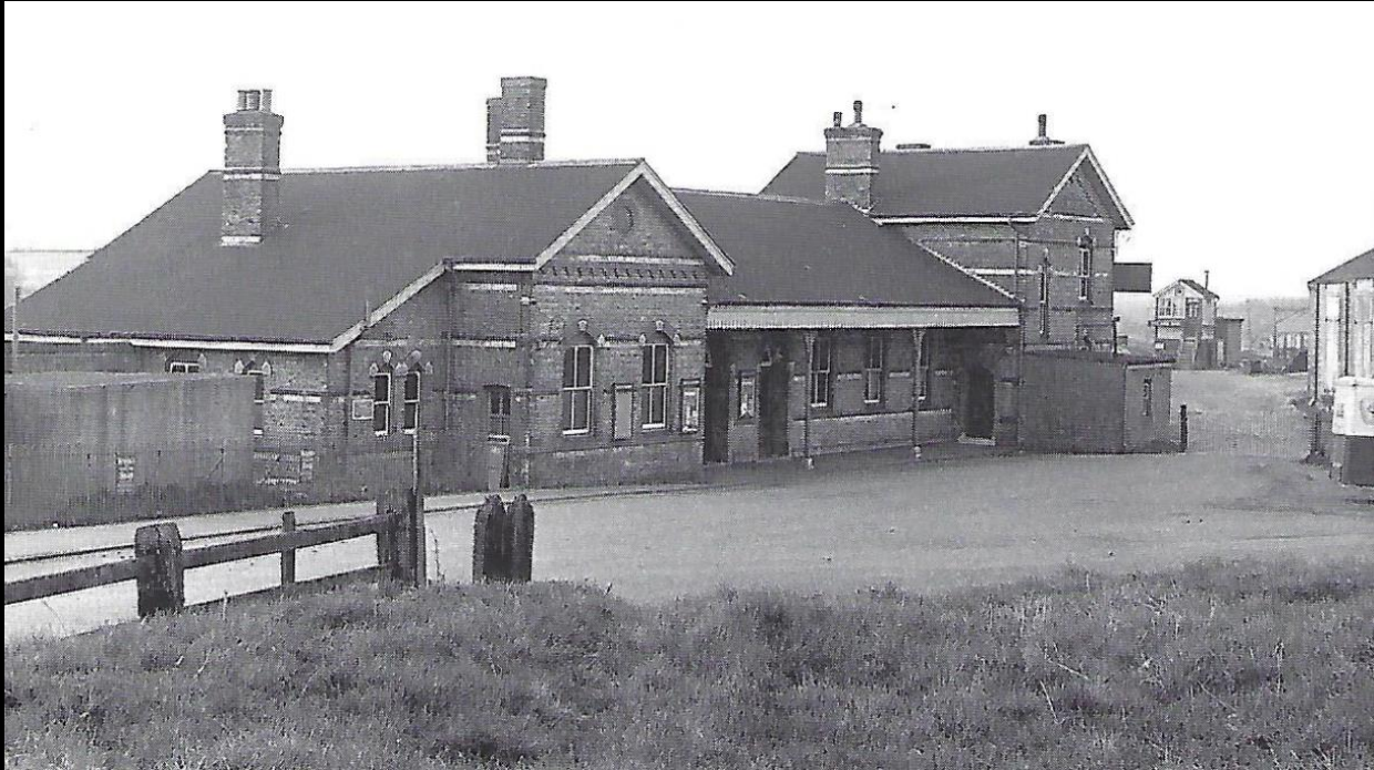
1960's – the bathroom extension has been added onto the station house
